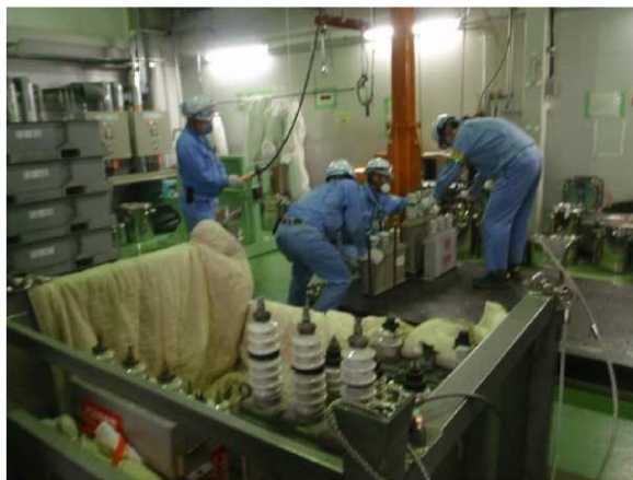
[H26.5.30 搬入状況の確認]
